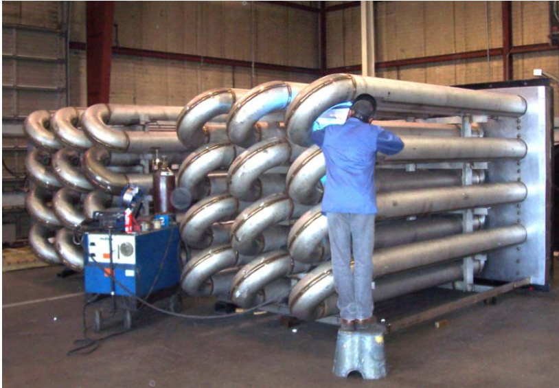
Figure #4. This picture shows the two burner plugs getting the last welding performed during fabrication.
