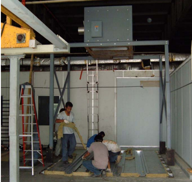
Figure 9: Heater box was raised and the insulated floor assembled.
